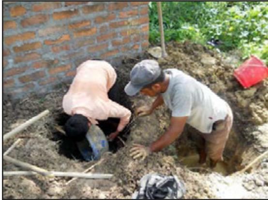
Figure a: Water pipe connecting to B2 bucket
